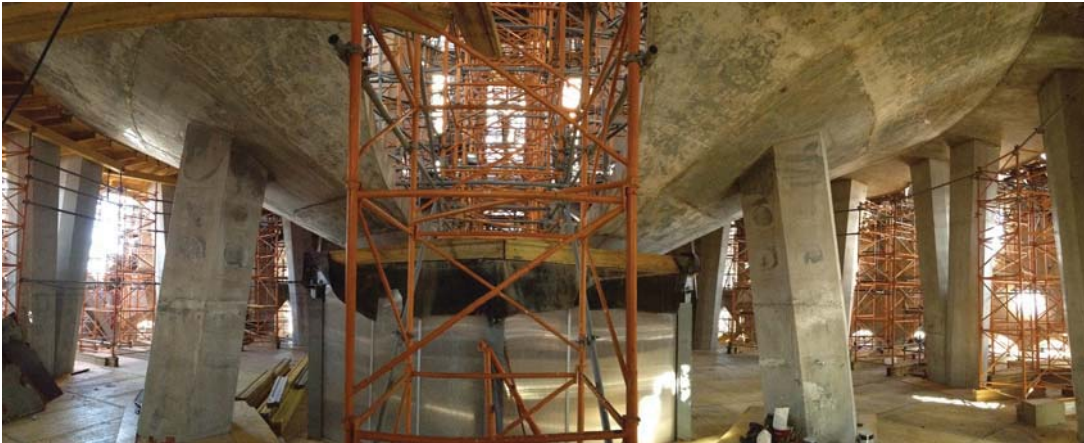
FIGURE 26.14 Undercroft of the auditorium.
