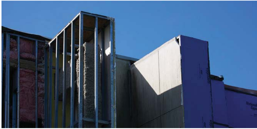
FIGURE 14.4 Metal stud wall surrounding projecting structural columns on the north façade.
