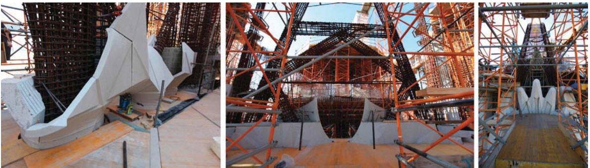
FIGURE 26.12 Permanent formwork with robot cut stone for exterior (LHS) and artificial stone on the interior (left); window nearing completion (middle); top of central window seen from the interior (right).
