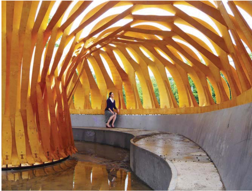
FIGURE 16.2 ICD/ITKE Research Pavilion 2010.
