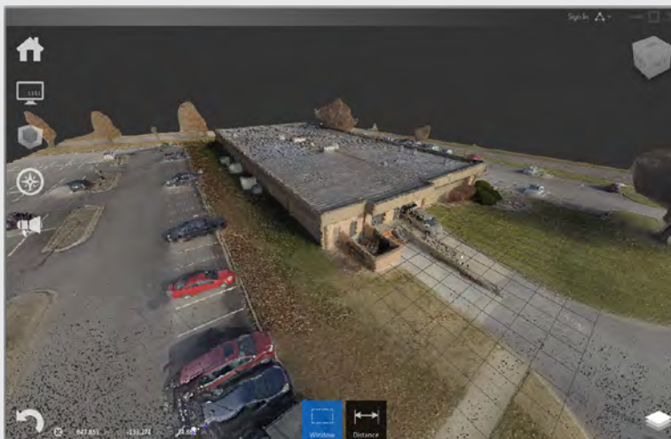
IMAGE COURTESY OF BLACK & VEATCH ENGINEERING
