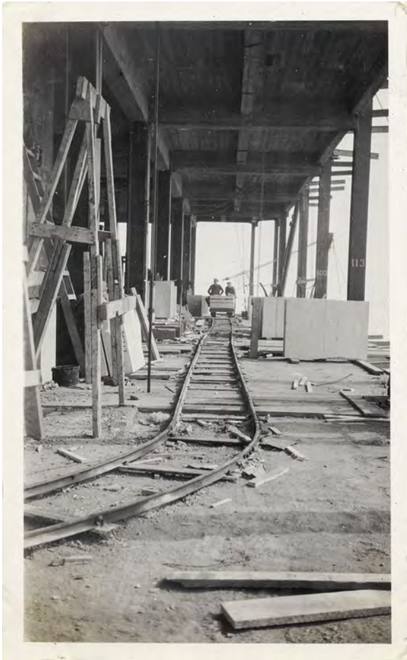
Figure 4.2 Industrial track (12 lb., 26-gauge rail) on 85th floor
