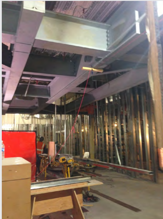
IMAGE COURTESY OF MCCARTHY BUILDING COMPANIES, INC.
