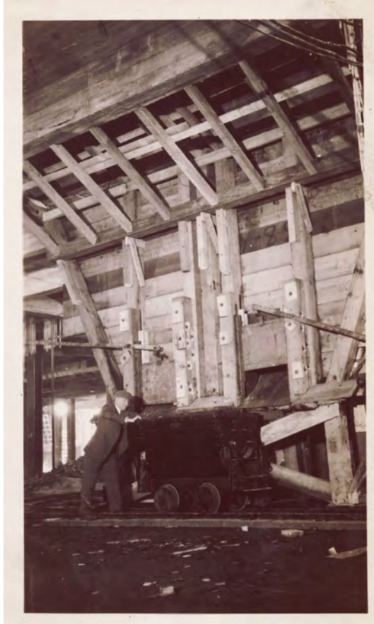
Figure 4.3 A Koppel rocker dump car on the track to the brick hopper
