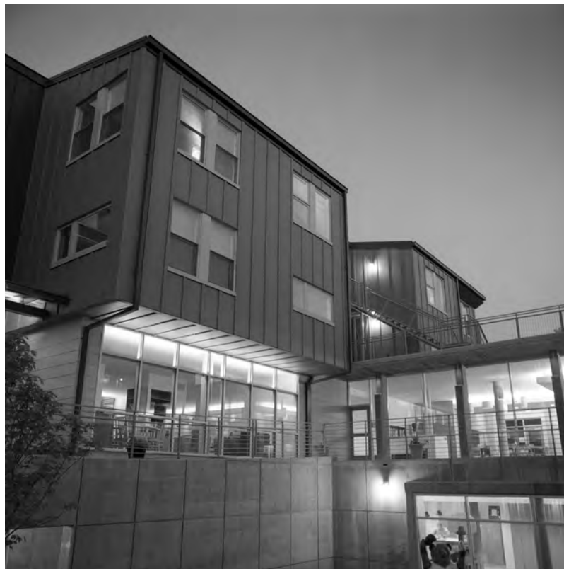
Figure 8.4 Ronald McDonald House built using BIM and prefabricated mockups
