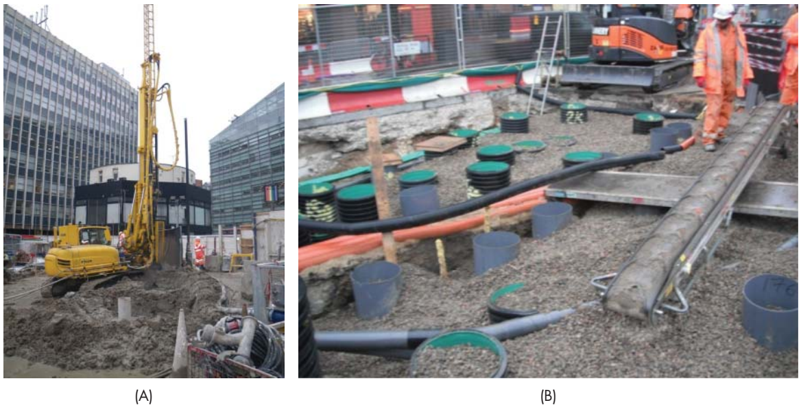
FIGURE 10–6–6 (A and B) Jet grouting at Victoria.
