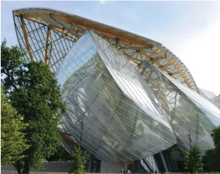
FIGURE 10-3-3 Free-form use of glass in the sails of the Fondation Louis Vuitton.
