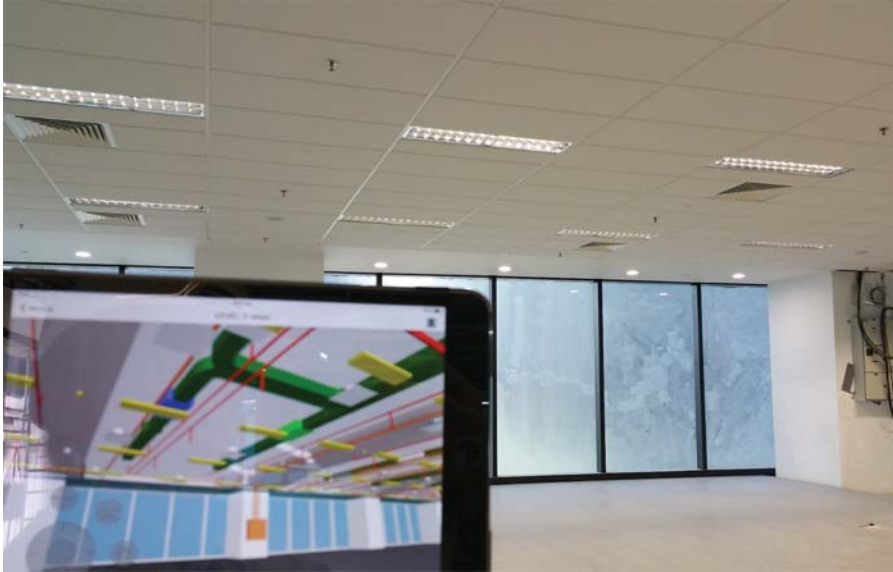
FIGURE 10–8–17 Detecting routing of concealed services with the as-built BIM model on iPad.
