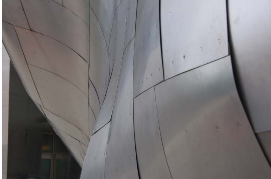
FIGURE 10-4-4 Intended gaps between panels at EMP, Seattle.
