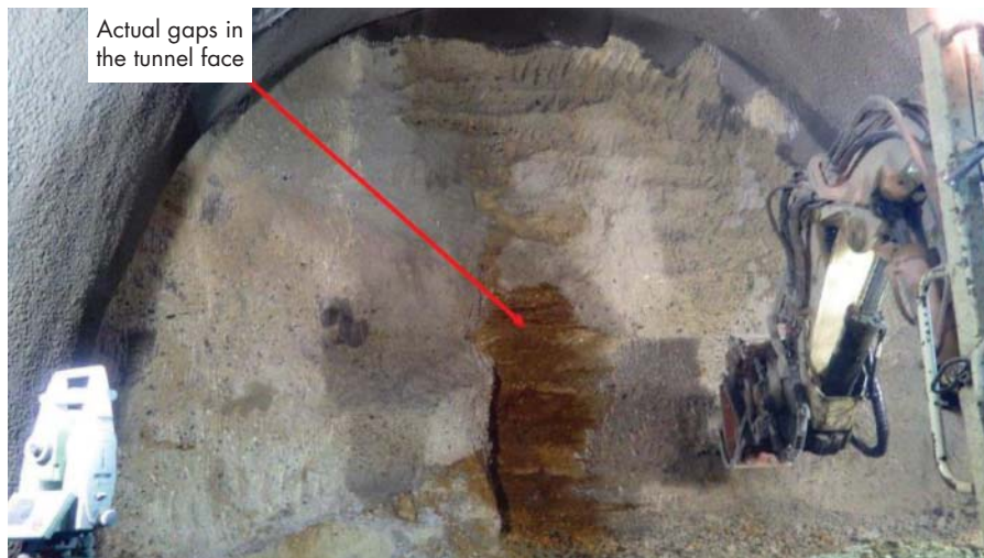
FIGURE 10–6–9 The same area of the jet grouting during excavation.
