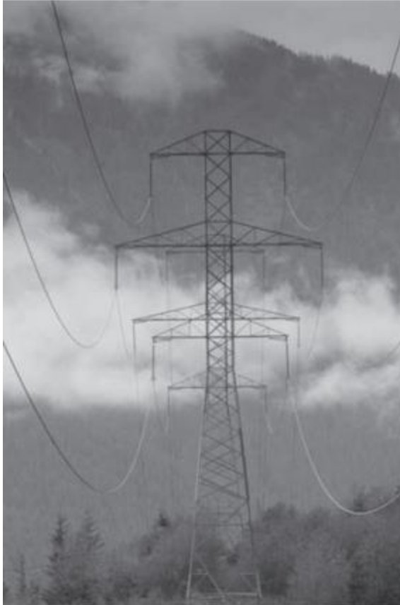
FIGURE 4.6: Suspension tower
